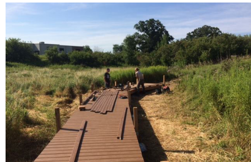
Photo of Boardwalk construction at landfill
