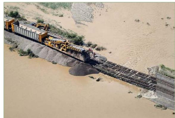
Figure 15: Crews work to repair washout damage near Stoddard, August 29, 2018. Source: Erik Daily, La Crosse Tribune.
