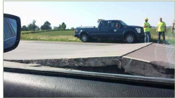
Figure 10: One of several “blow-ups” that occurred along I-90 in Minnesota in June 2016. Source: Minnesota Department of Transportation.
