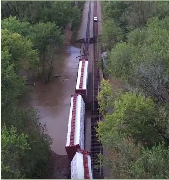
Figure 16: Derailed BNSF train from washout of bridge over Rush Creek south of Ferryville, WI, September 22, 2016. Source: Snapshot from YouTube video, DOT-111.info.
