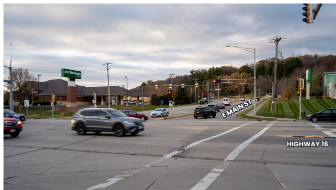
Figure 28. Highway 16 & N Kinney Coulee Rd/E Main St Existing Conditions
