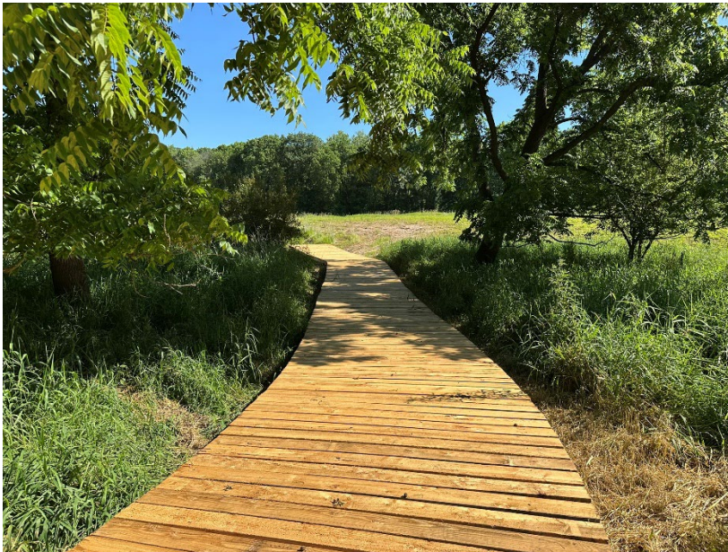
Figure 4.31. Mixed use trail under construction.
