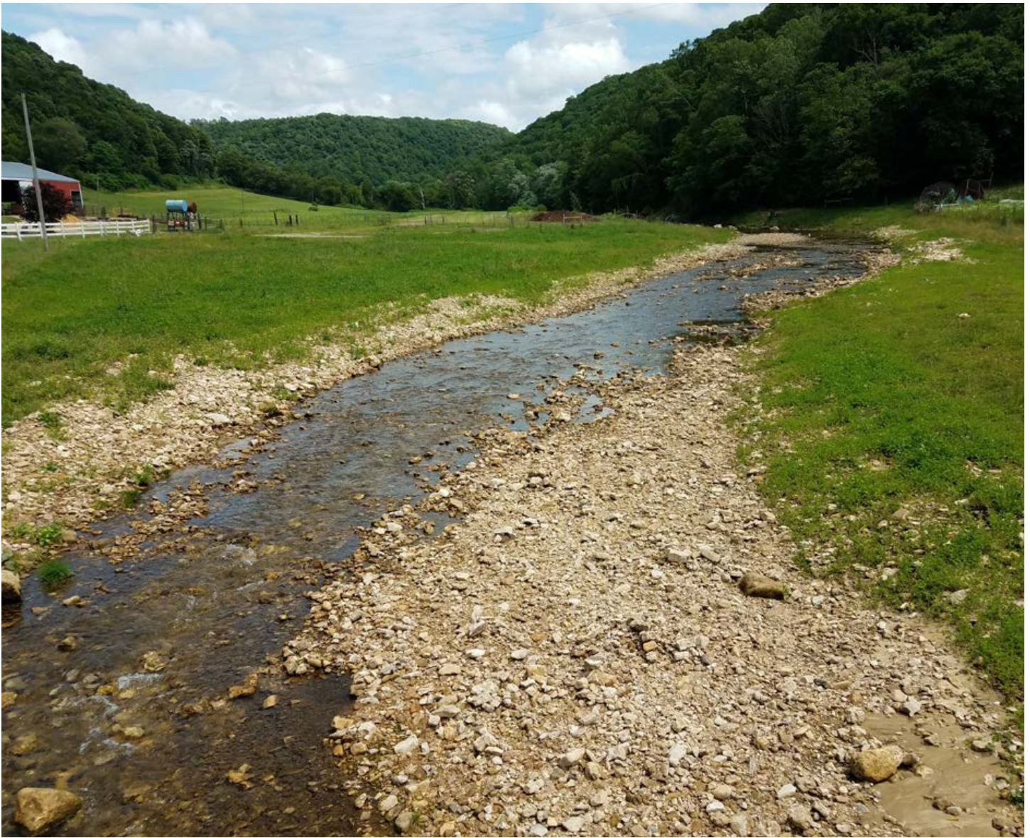
Stream reach in the Rullands Coulee sub-watershed within the Coon Creek Watershed that was impacted by upstream dam breaches in 2018. Photo by Eric Booth
