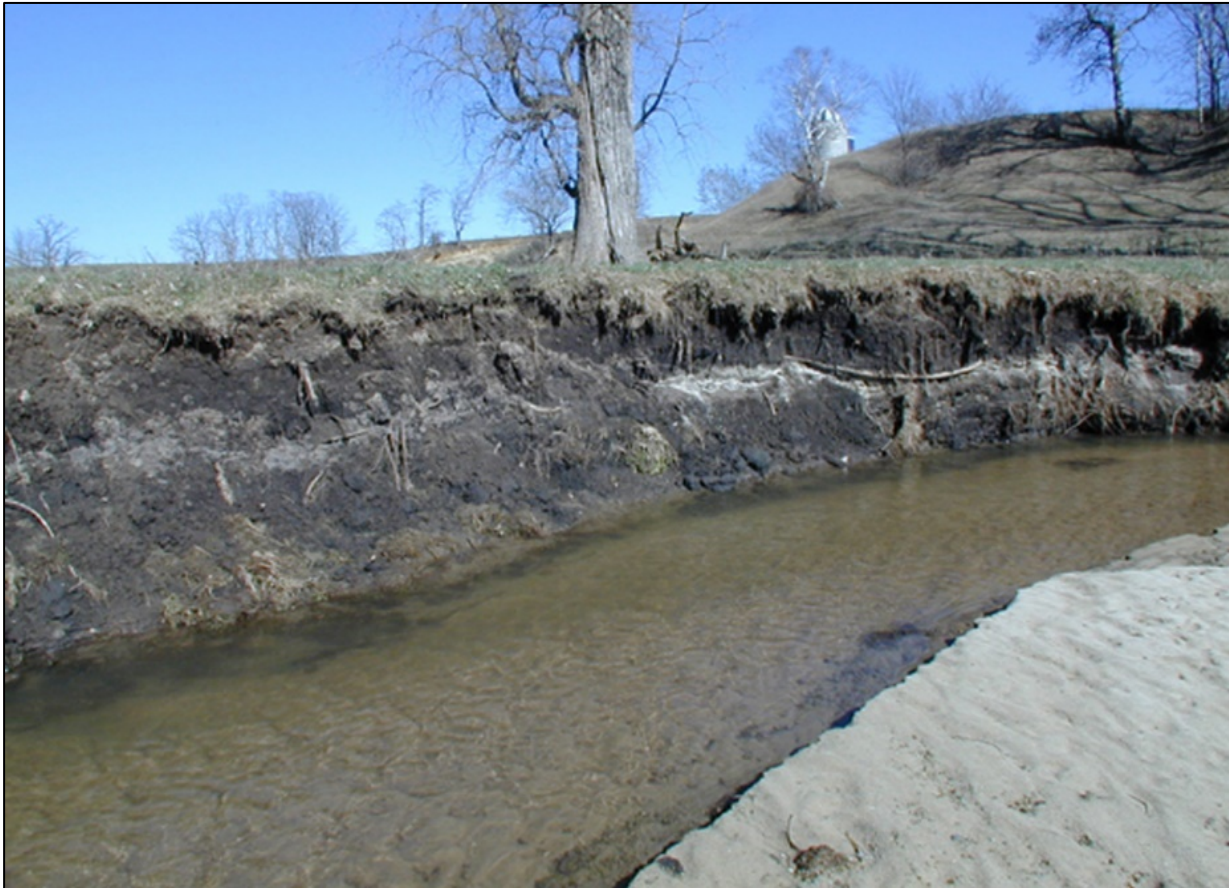
Figure 18 Streambank Erosion Photo
