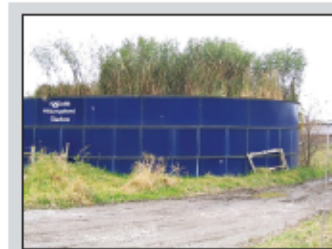
Abandoned waste storage structure.
