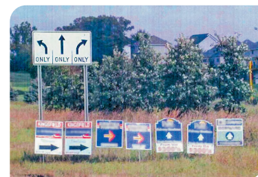
Improperly placed signs can add to the clutter along the roadside and be confusing to motorists.
