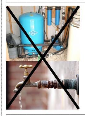
**Step 2:** <u>DO NOT</u> use the pressure tank sampling tap, an outside tap or laundry tub faucet. These fixtures are constructed of brass which contains lead and copper. Corroded brass will flake off during sampling and cause falsely high results.
