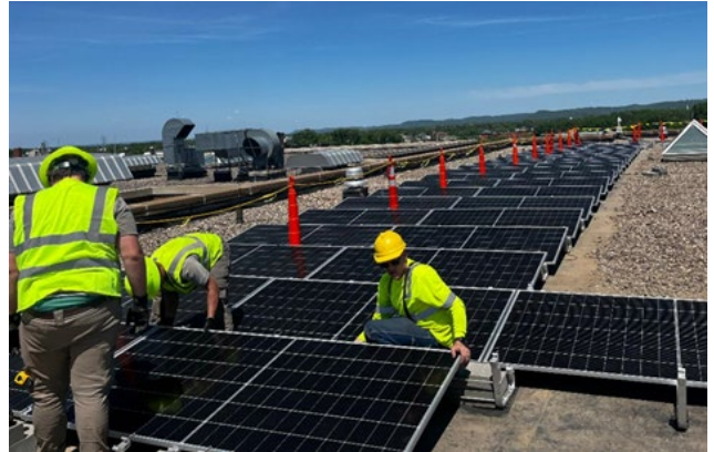
Figure 3. A solar photovoltaic energy system being installed at the County Law Enforcement Center May 2024.
