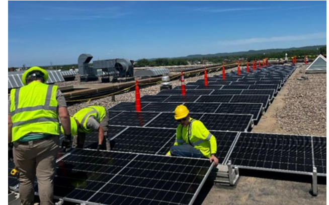
Figure 20. A solar photovoltaic energy system being installed at the LCC Law Enforcement Center May, 2024.
