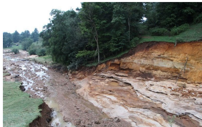
Figure 8. Aftermath of a 2018 earthen dam break due to heavy rain events in Monroe County. Source: LaCrosseTribune.com
